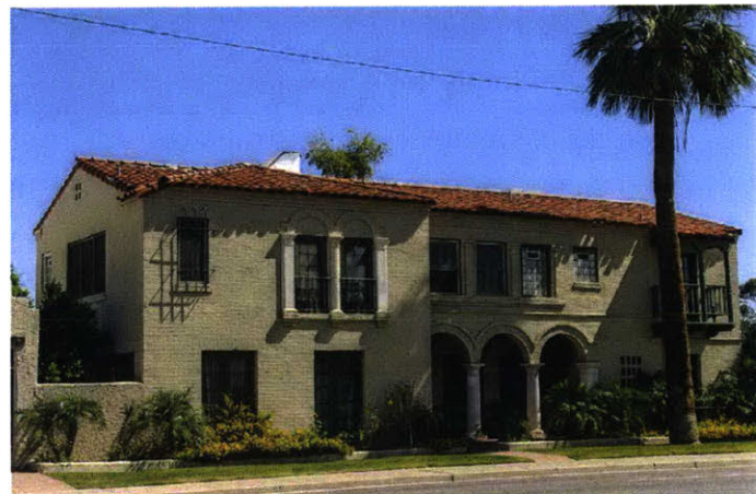
Figure 2.7: Multiplex: Small ( Missing Middle, 2017 )
