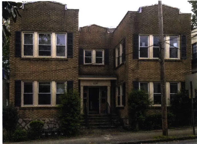
Figure 2.6: Fourplex ( Missing Middle, 2017 )
