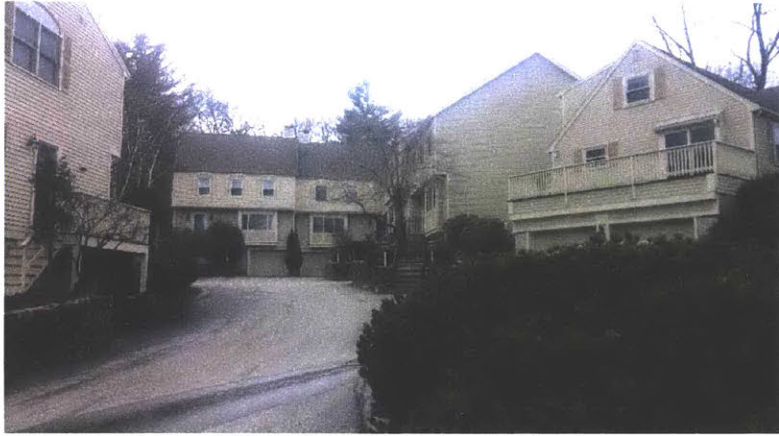
Figure 4.21: Wellesley's housing: Small multiplex
