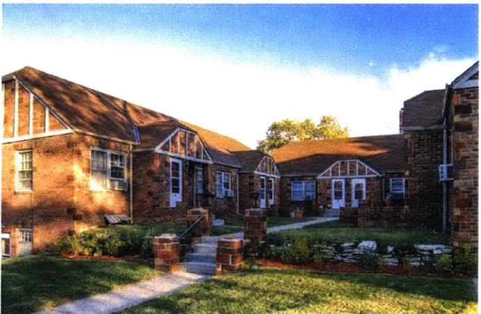
Figure 2.10: Courtyard Apartments ( Missing Middle, 2017 )
